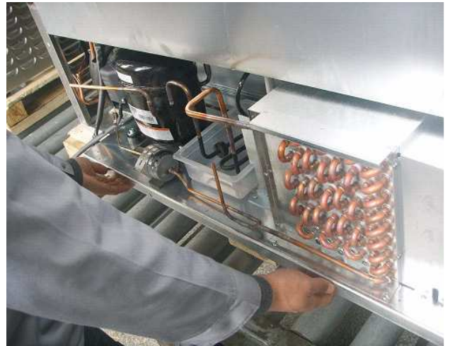
Pull out the condensing unit
